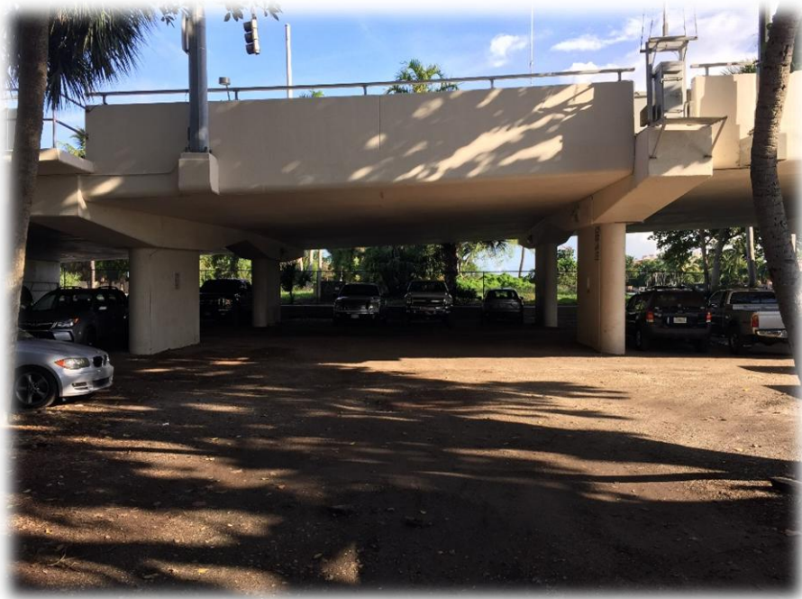
Figure 2 Under bridge linkage from Silver Palm Park to The Wildflower
